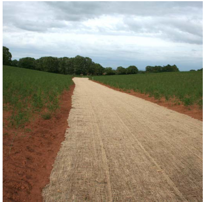
Figure 3. Bespoke GWW with jute geotextile to provide immediate protection from rainfall and runoff
