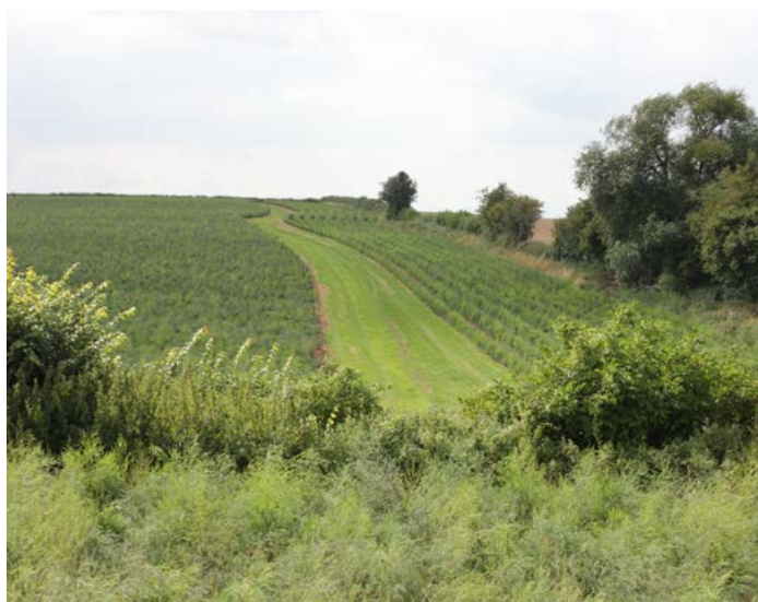
Figure 5. Grassed waterways are designed to sit within the natural topography with minimum land engineering.
